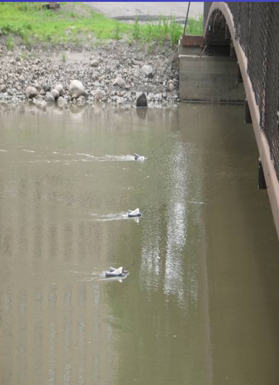
Oak Grove Steel Bridge
