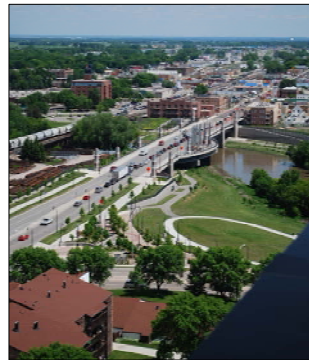
Main Street Bridge
