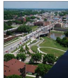
Main Street Bridge
